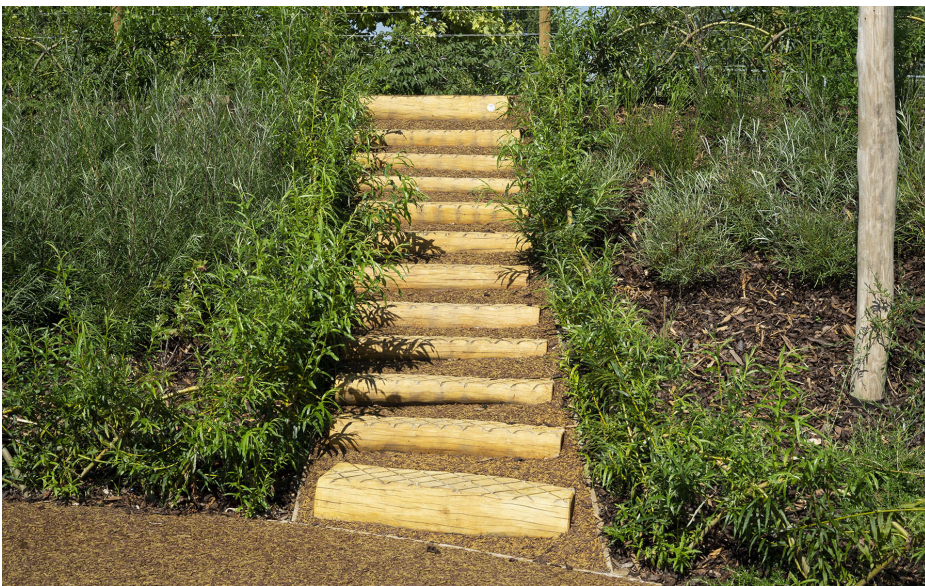
Timber steps, set in Tiger Mulch play safety surface
